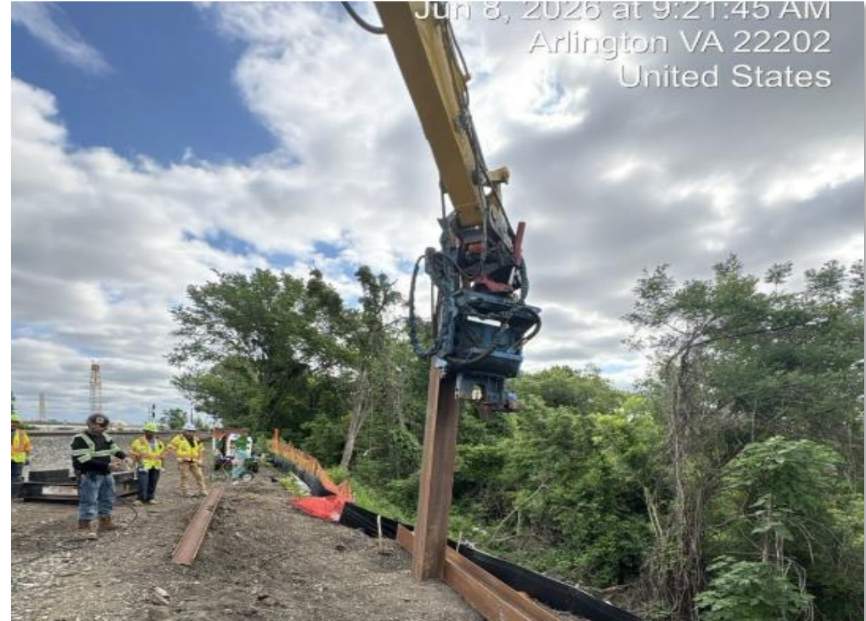
Pile driving at Crystal City
