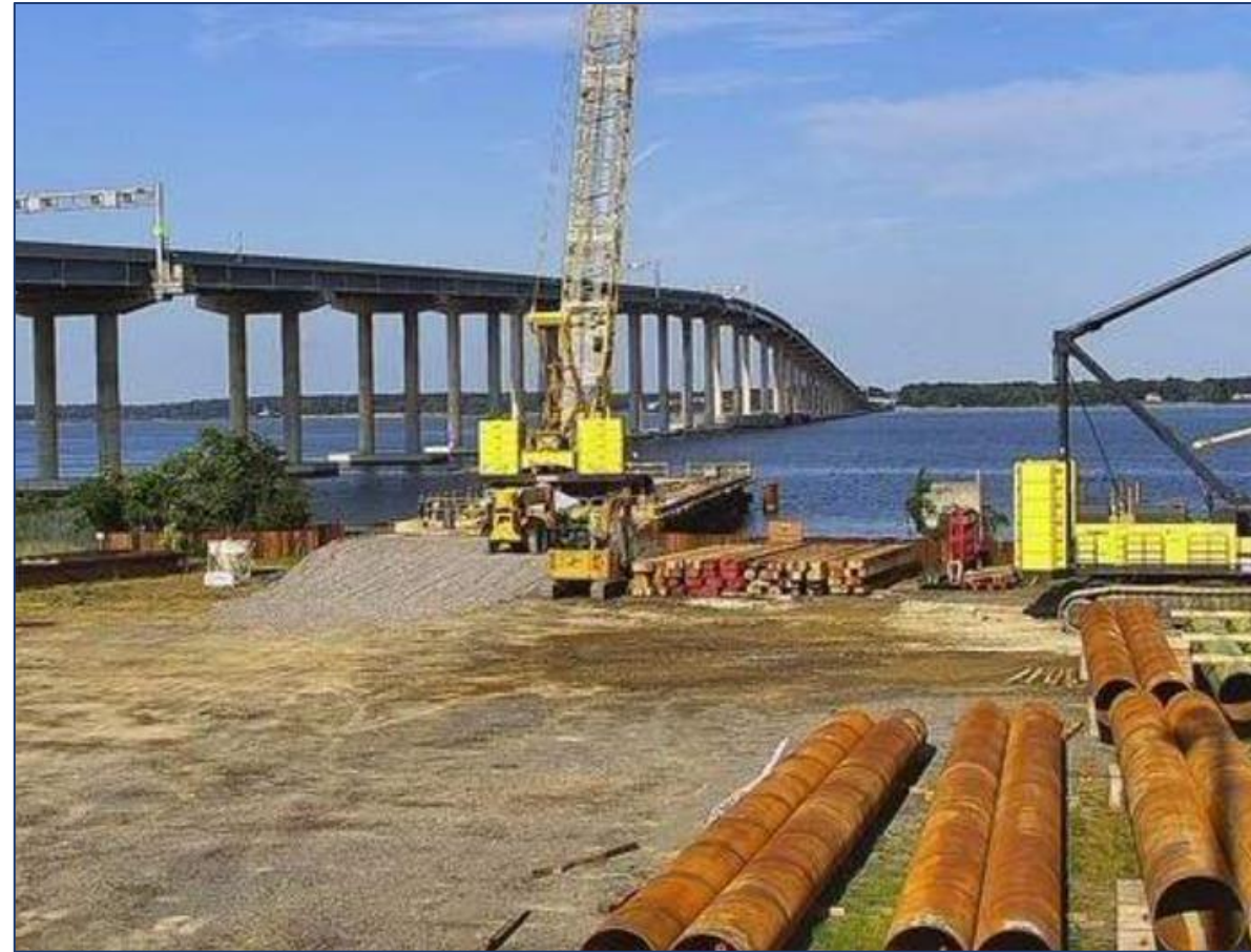
Harry Nice Bridge Trestle Material Staging Area
