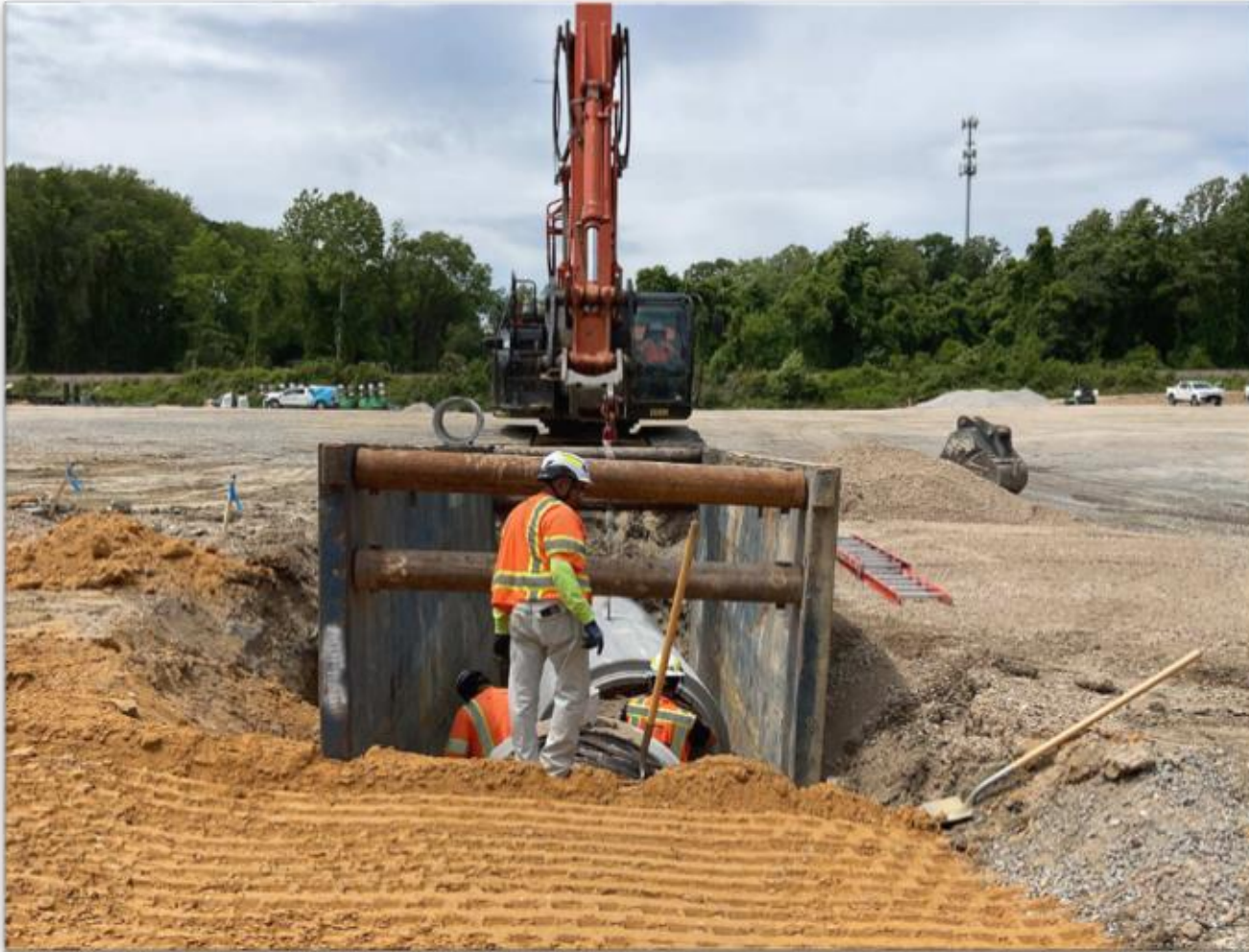
Stormwater drainage installation
