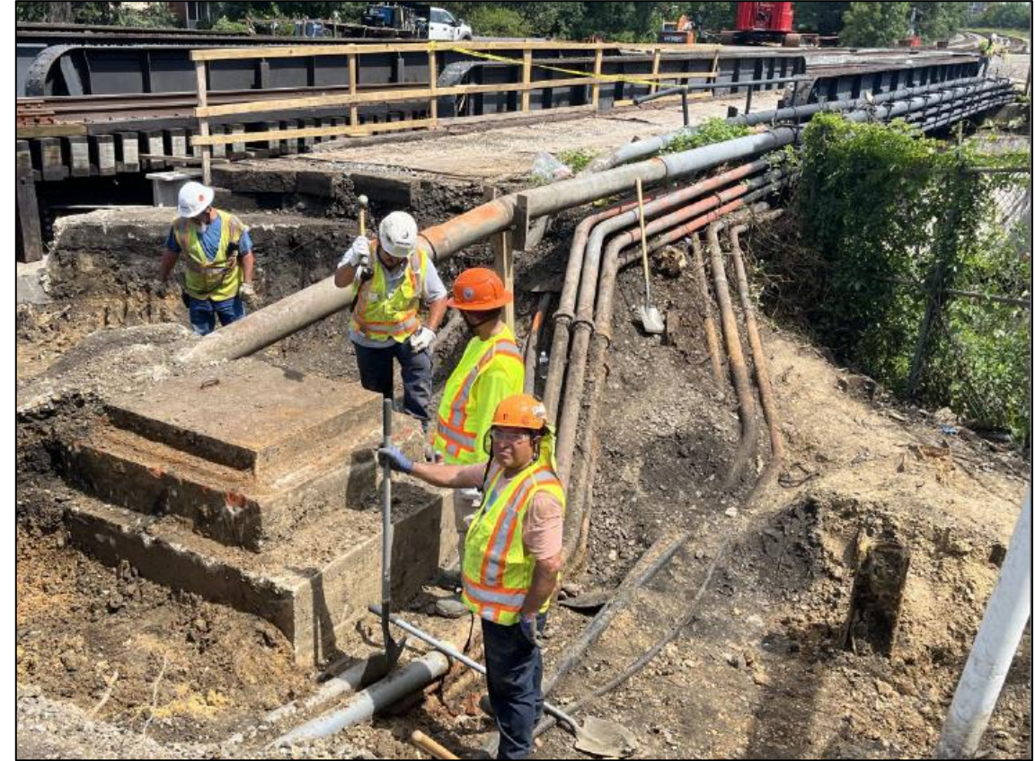
Fiber utility relocation
