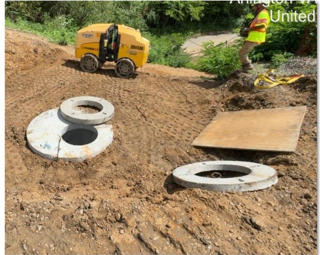
Drainage structure installation
