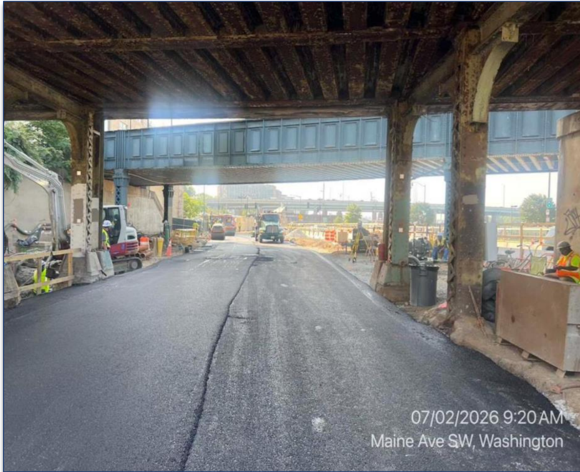
Maine Ave. Maintenance of Traffic Crossover
