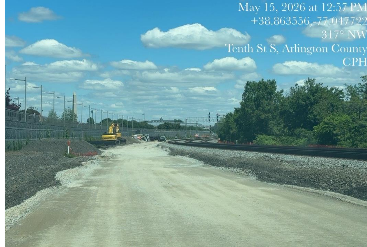
Grading at MP 109 on Track 1
