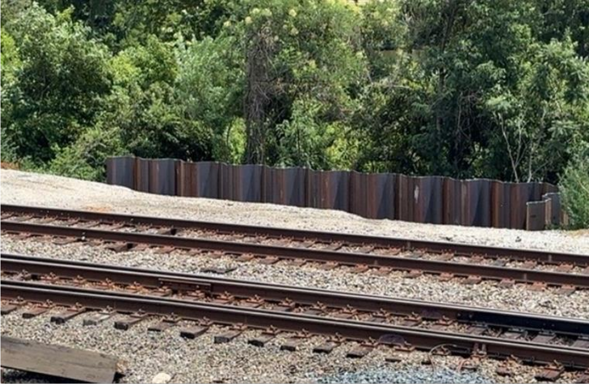
Completed Retaining Wall at Milepost 109.7
