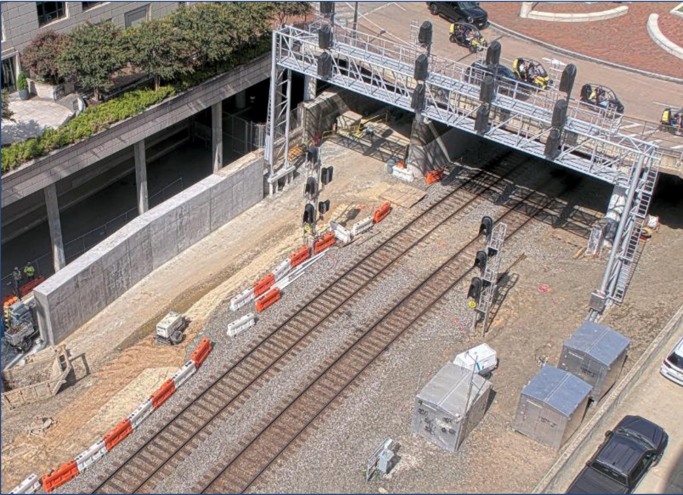
Retaining Wall L Cast-in-place & new CSX Signal Bridge
