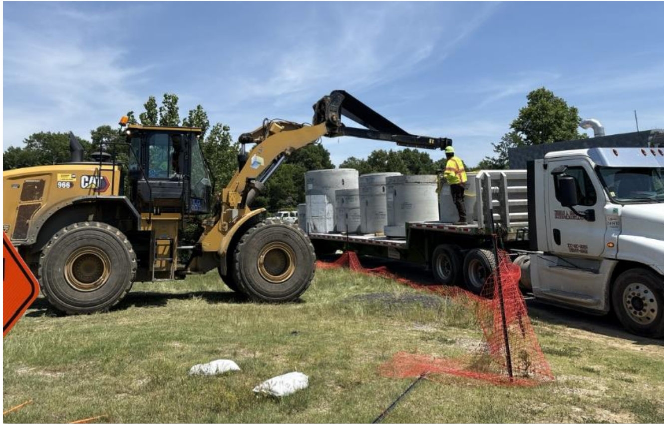
Material delivery & unloading
