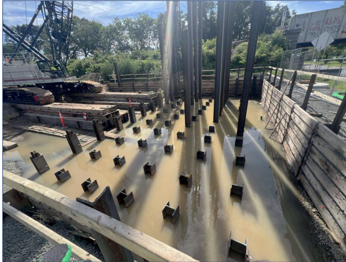
Abutment B (DC) pile driving
