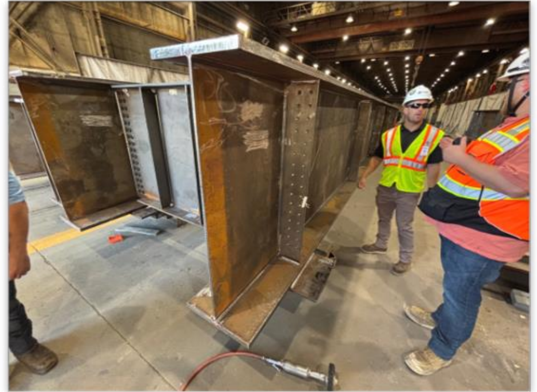
Off-site structural steel fabrication
