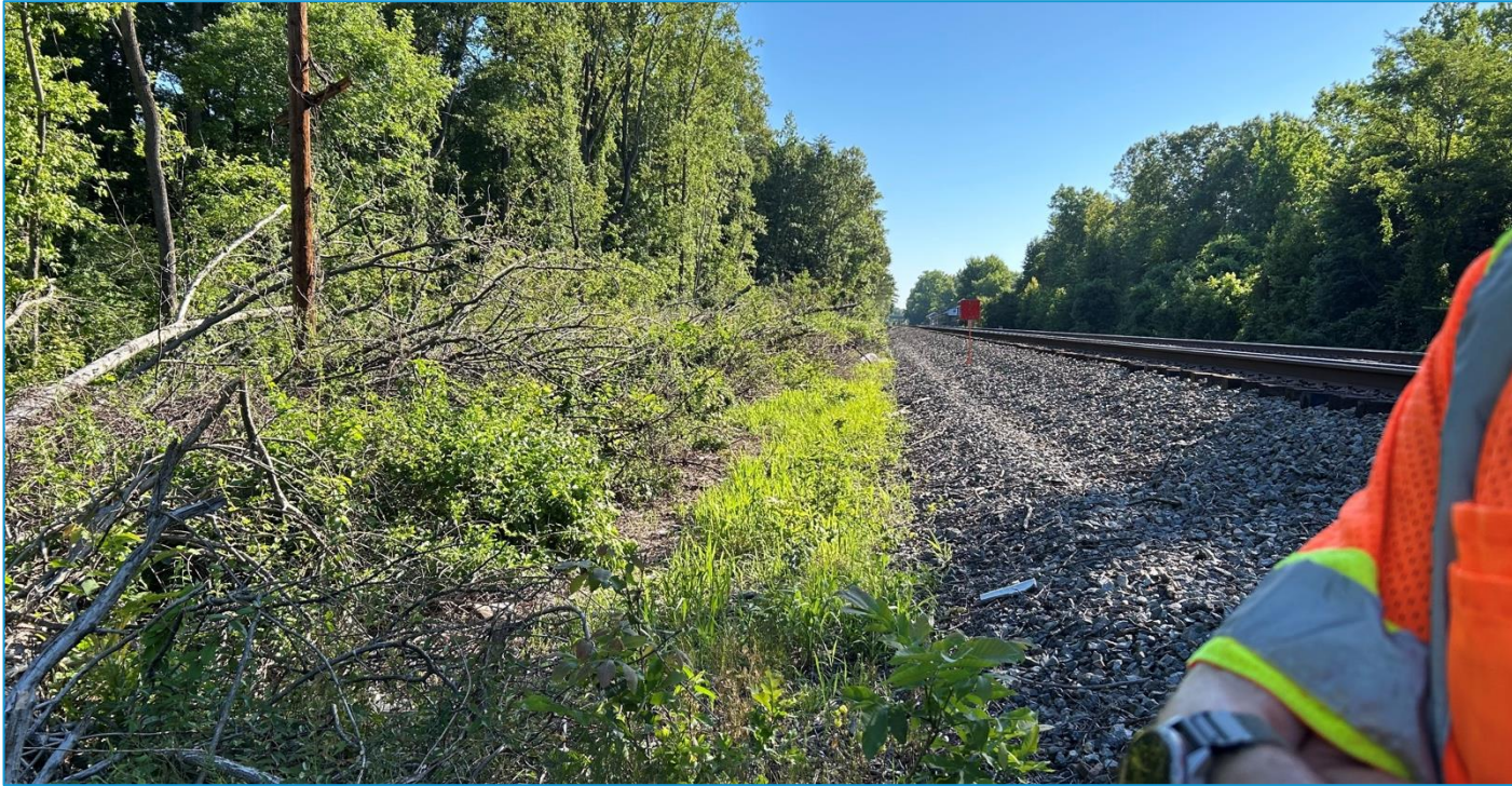
Tree Clearing for Fairfax Sewer Relocation
