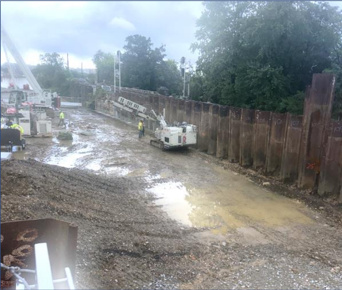
Abutment A (VA) Support-of-Excavation installation adjacent to CSX tracks
