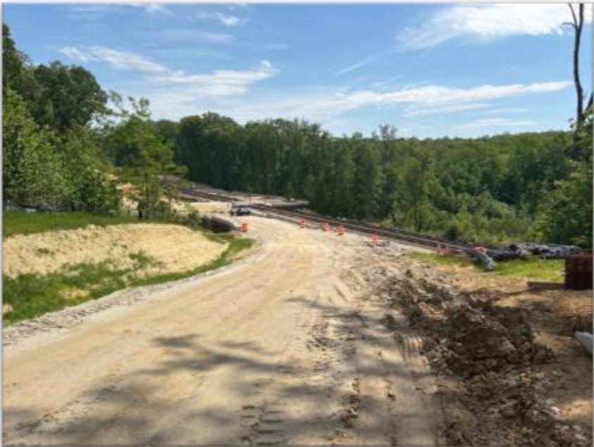
Loisdale Road site access
