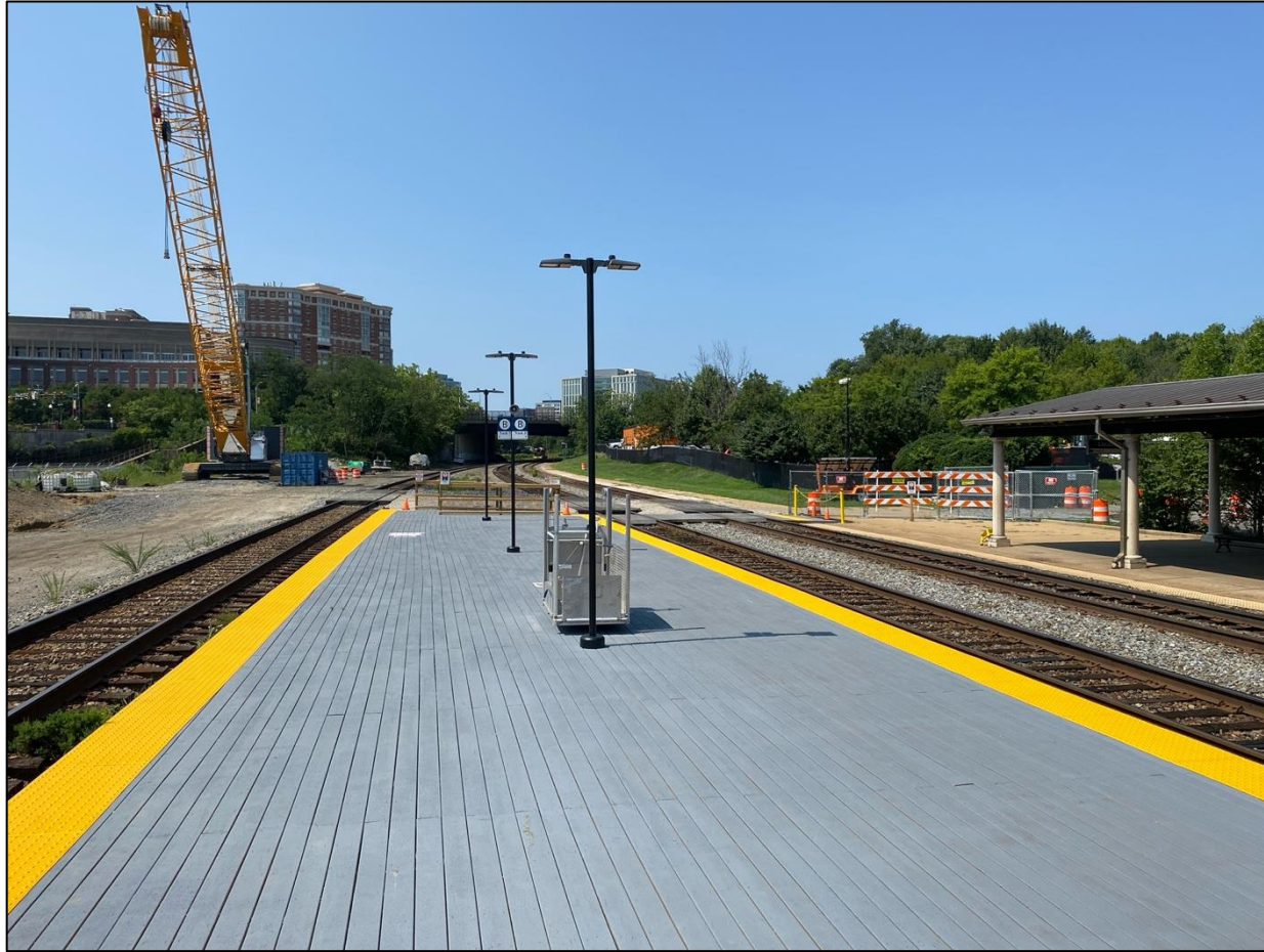
The temporary platform serving Tracks 1 and 2 was extended with a new pedestrian crossing to the station.
