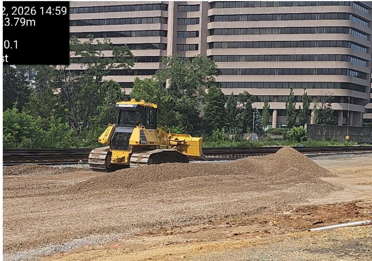
Sub-ballast installation for future fourth track
