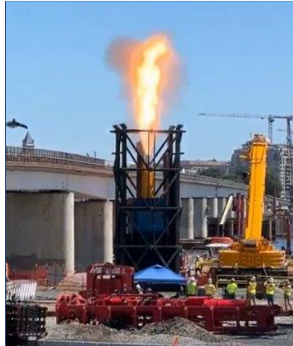
Statnamic Test on 24" VA Land Pile
