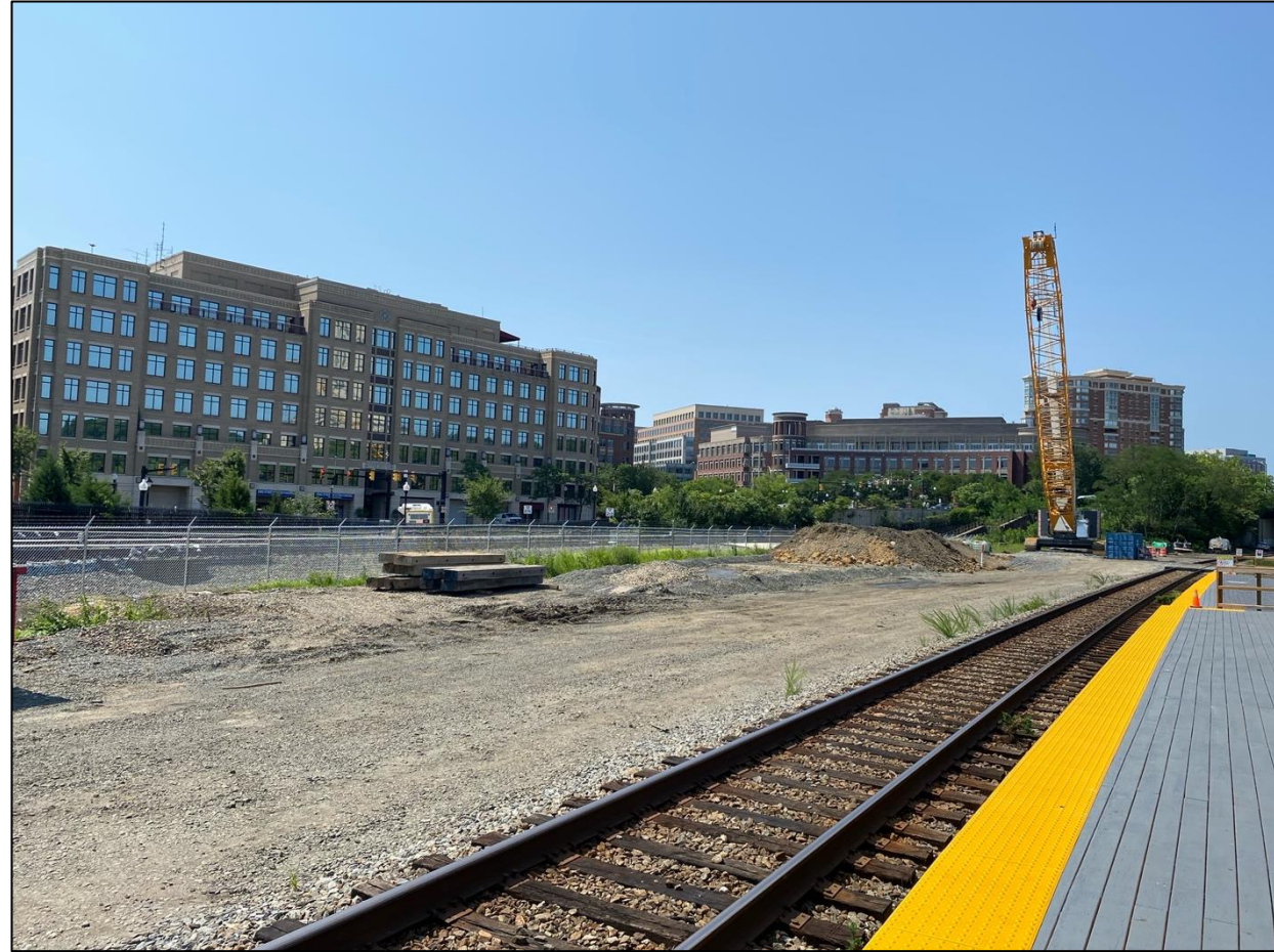
The metro station intrusion-detection fence was relocated.
