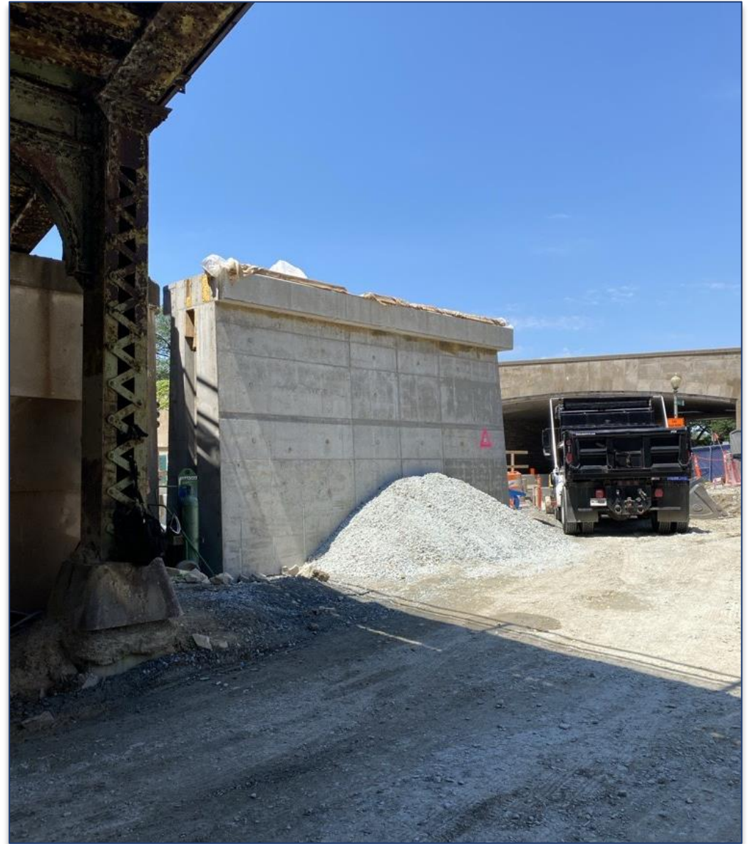
Maine Ave. Bridge Pier 2
