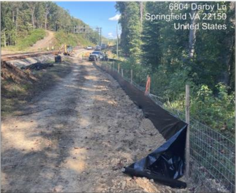
Erosion and Sediment Controls being Installed
