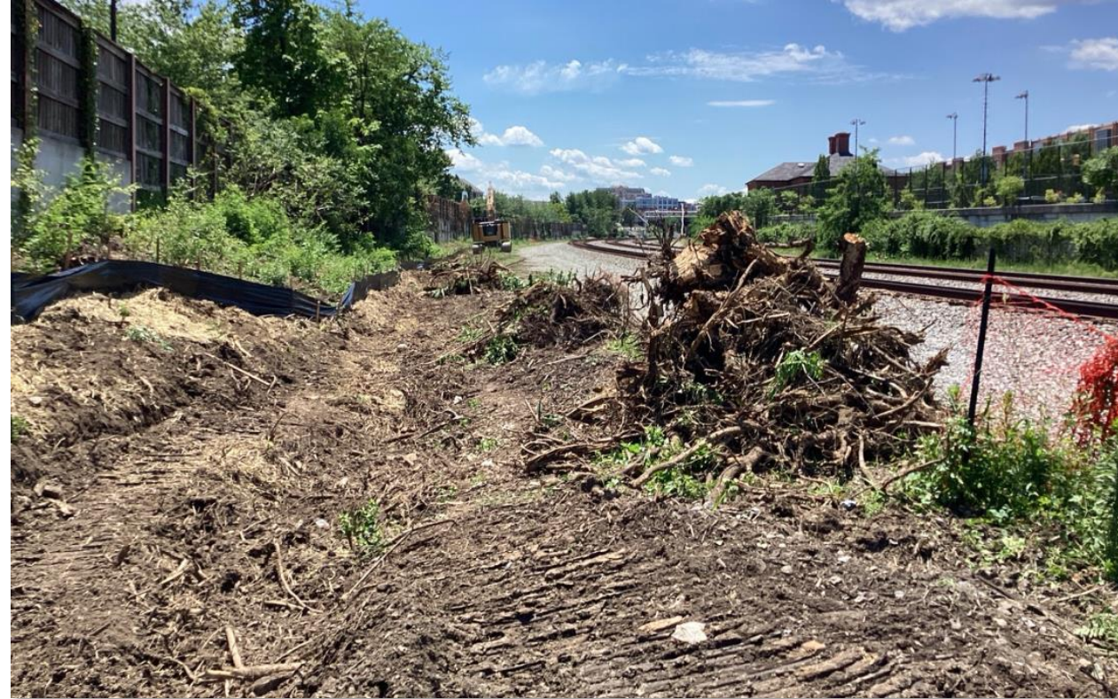
Clearing & grubbing at Potomac Greens
