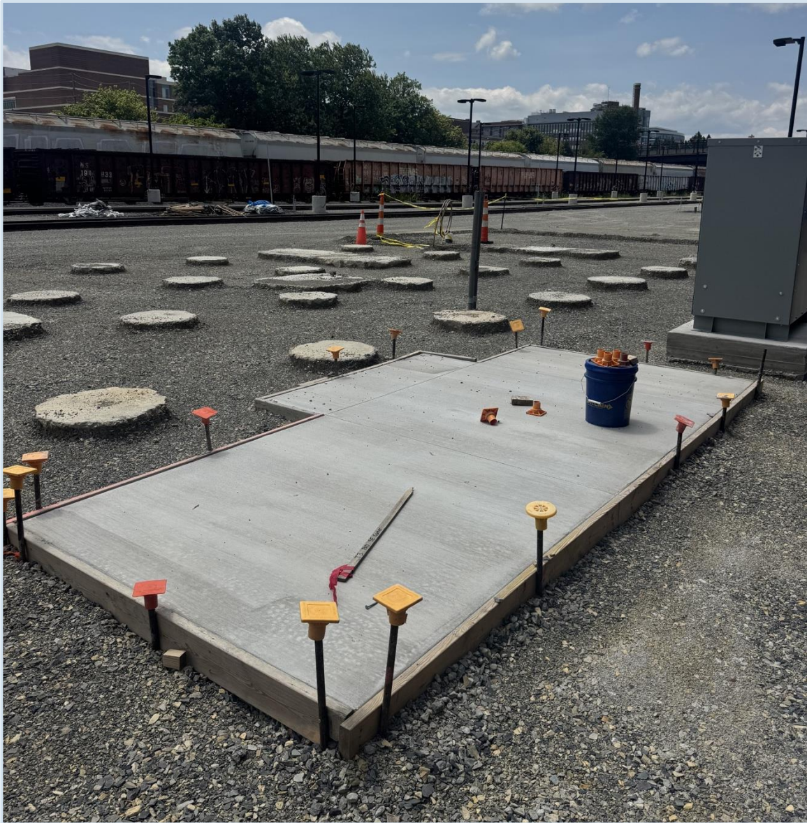
Foundations for modular building
