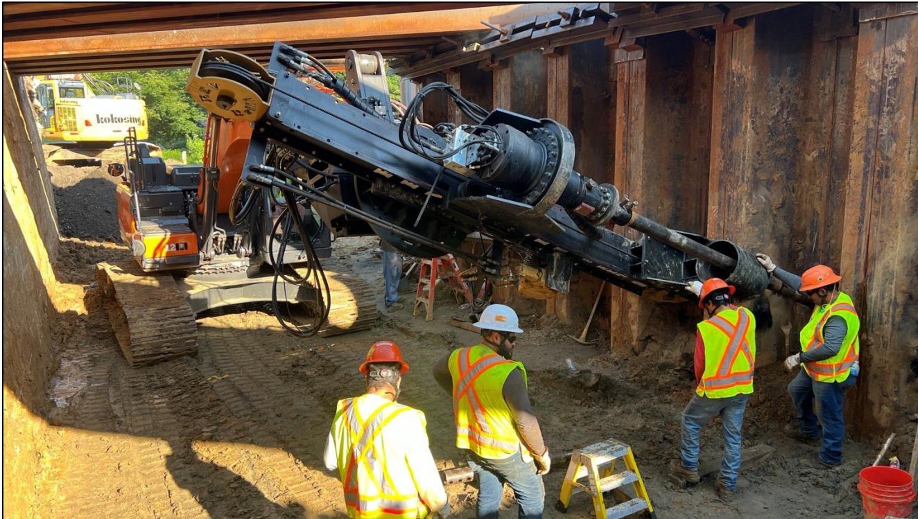
Helical anchors installation
